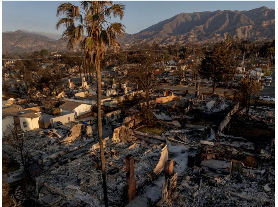
Eaton Canyon, CA - Homes after the Eaton Fire in 2025.
